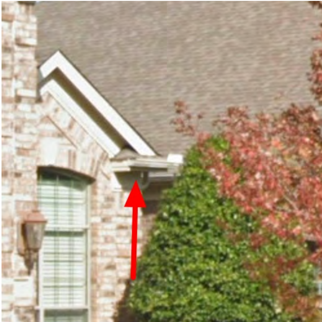
9 Gable cornice return
